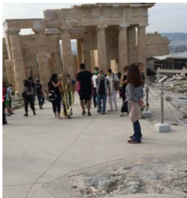
New pathway at the Athens Acropolis made of a specific concrete to provide a smooth and non-slippery surface. ©Katerina Papamichail
